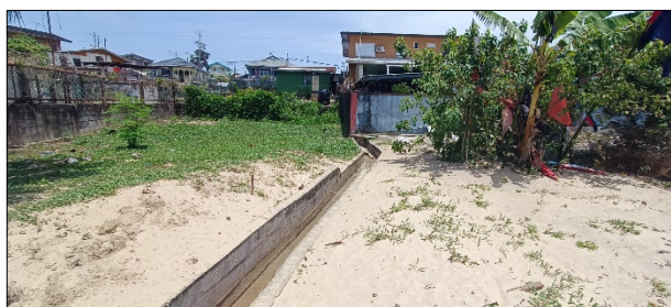
Photos 31 and 32. Presence of concrete micro-dumping sites and gullies on the beach that channel wastewater and runoff seaward. Central part of Sector 1.
