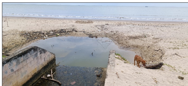
Photos 29 and 30. Presence of a concrete structure that channels wastewater and runoff seaward. East end of Sector 1.
