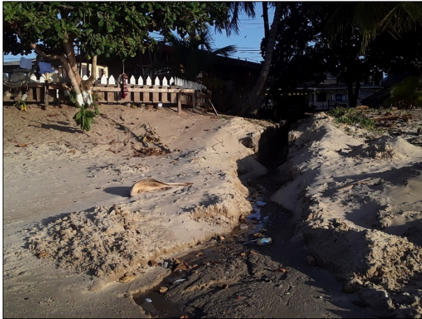
Photo 51. Sewage discharges through micro-dumps directly onto the beach.
