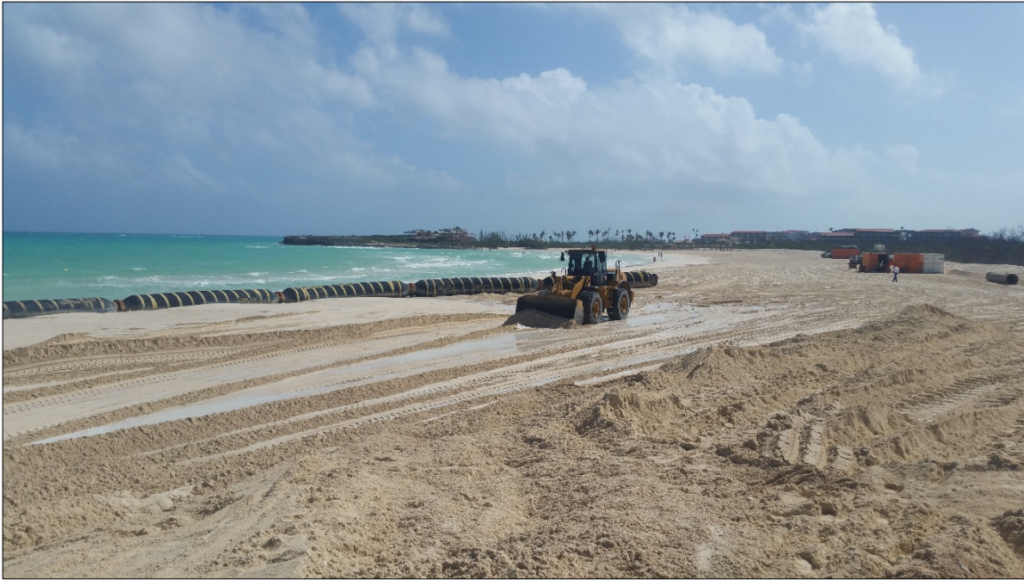
Photo 74. Leveling and shaping of the beach profile by mechanical equipment.
