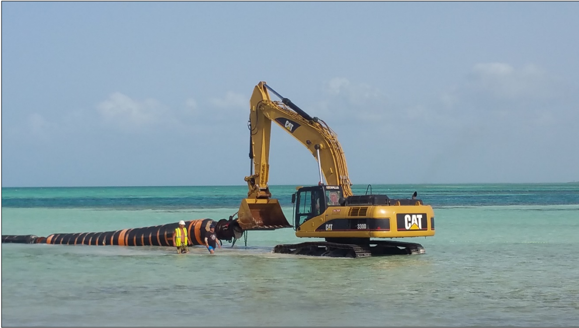
Photo 72. Backhoe placing the end of the pipe at the discharge point.
