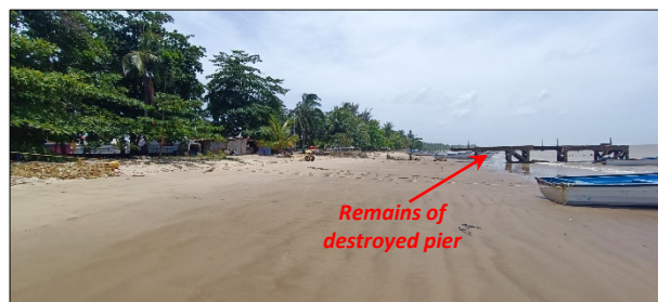
Photo 40. Remains of a destroyed pier that still rests on the beach.
