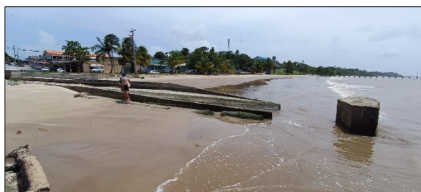
Photos 33 and 34. Presence of a concrete structure that channels wastewater and runoff seaward. West end of Sector 1.
