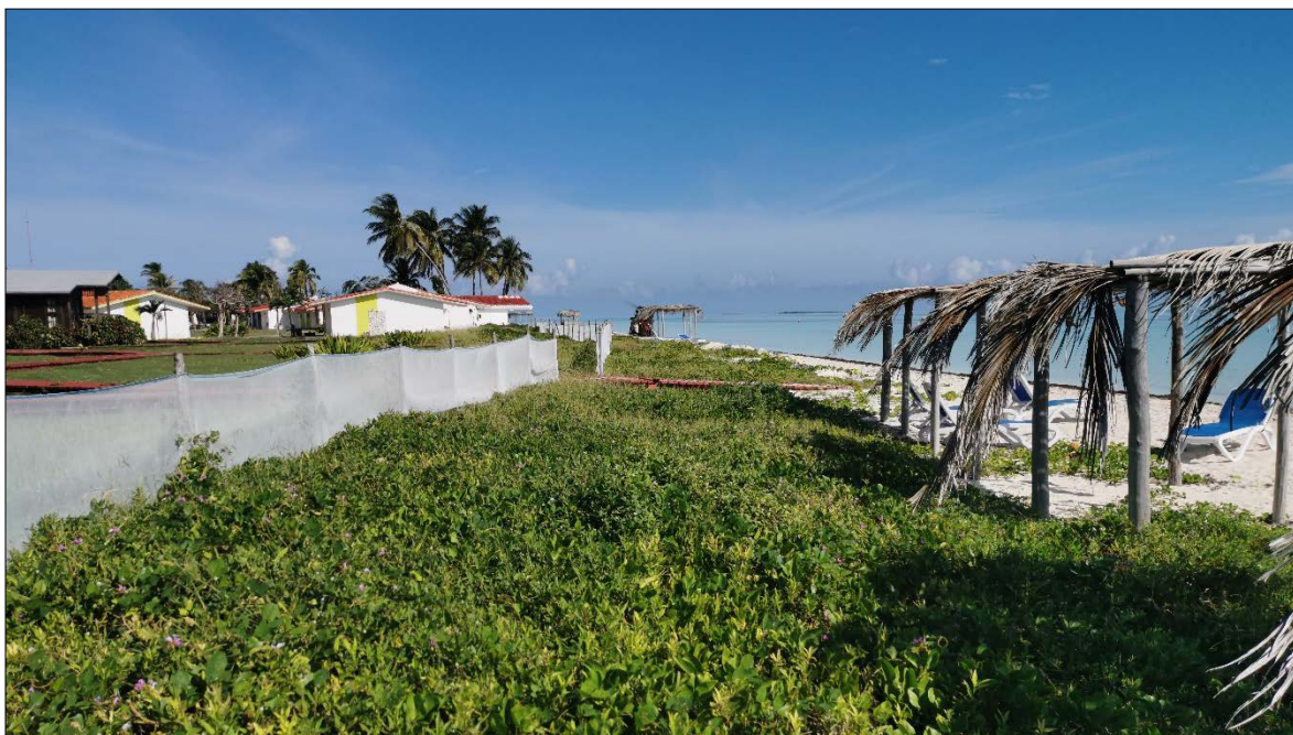
Photo 70. Containment barriers and sand catchment implemented in El Paso Beach, Cayo Guillermo, Cuba.
