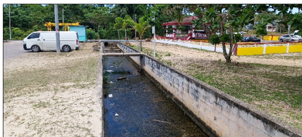
Photos 29 and 30. Presence of a concrete structure that channels wastewater and runoff seaward. East end of Sector 1.
