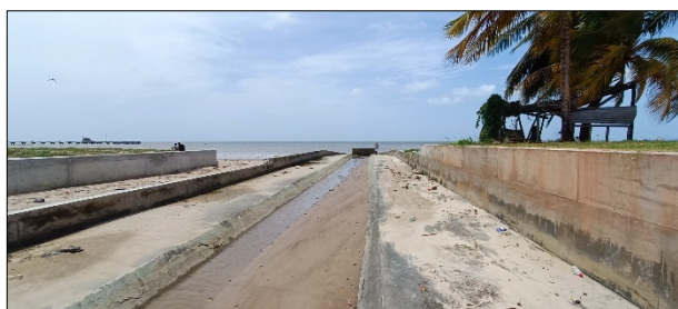
Photos 33 and 34. Presence of a concrete structure that channels wastewater and runoff seaward. West end of Sector 1.
